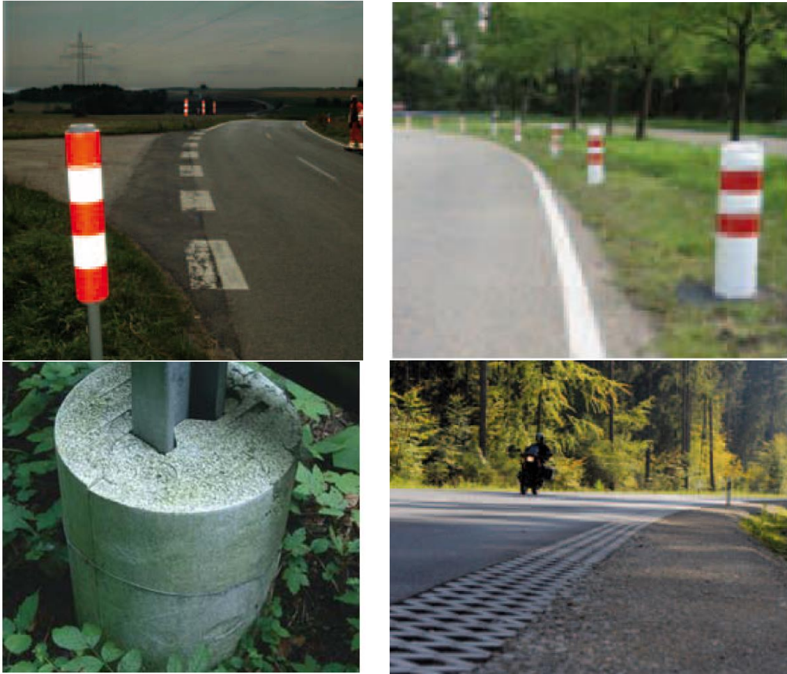
Figure 8. Some of the measures provided in the Slovenian specification in the road equipment phase; from upper-left: flexible bollards, flexible 'balisette' bollards, motorcycle collision shock absorbers and a reinforced shoulder between the pavement and the slope of the embankment
